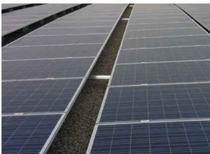
3 degree tilt improves array density with tighter row spacing
